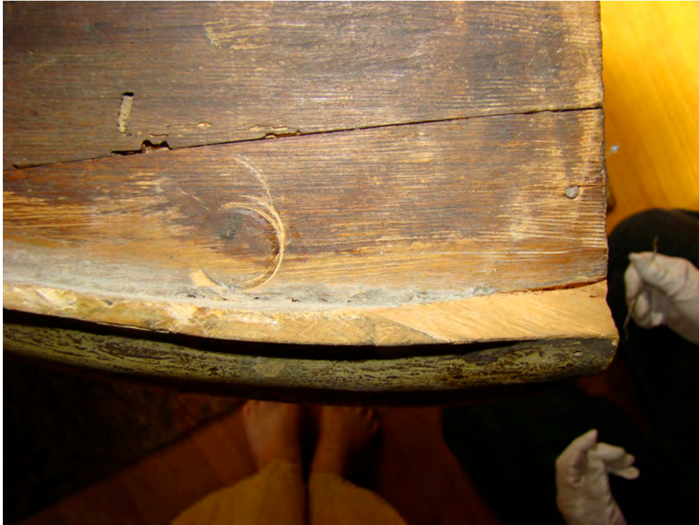
POLYCHROME ITALIAN CORNER CUPBOARD: BEFORE AND AFTER TREATMENT (NOTE THE C-CLAMP MARK FROM A SLOPPY PREVIOUS REPAIR.)
